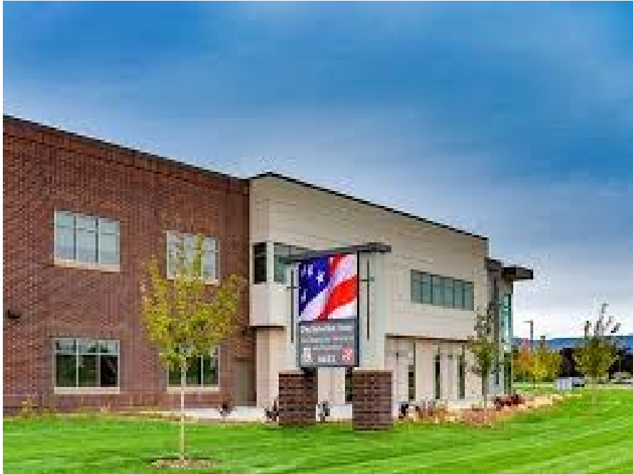
Street view of school from Emerald
