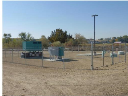
Franklin Pump Station
