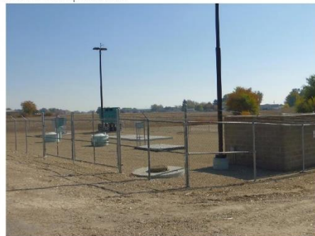
Franklin Pump Station
